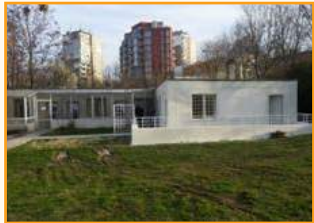
Early stages of Bulgaria SARC. Photo courtesy of Alison Eaton.
