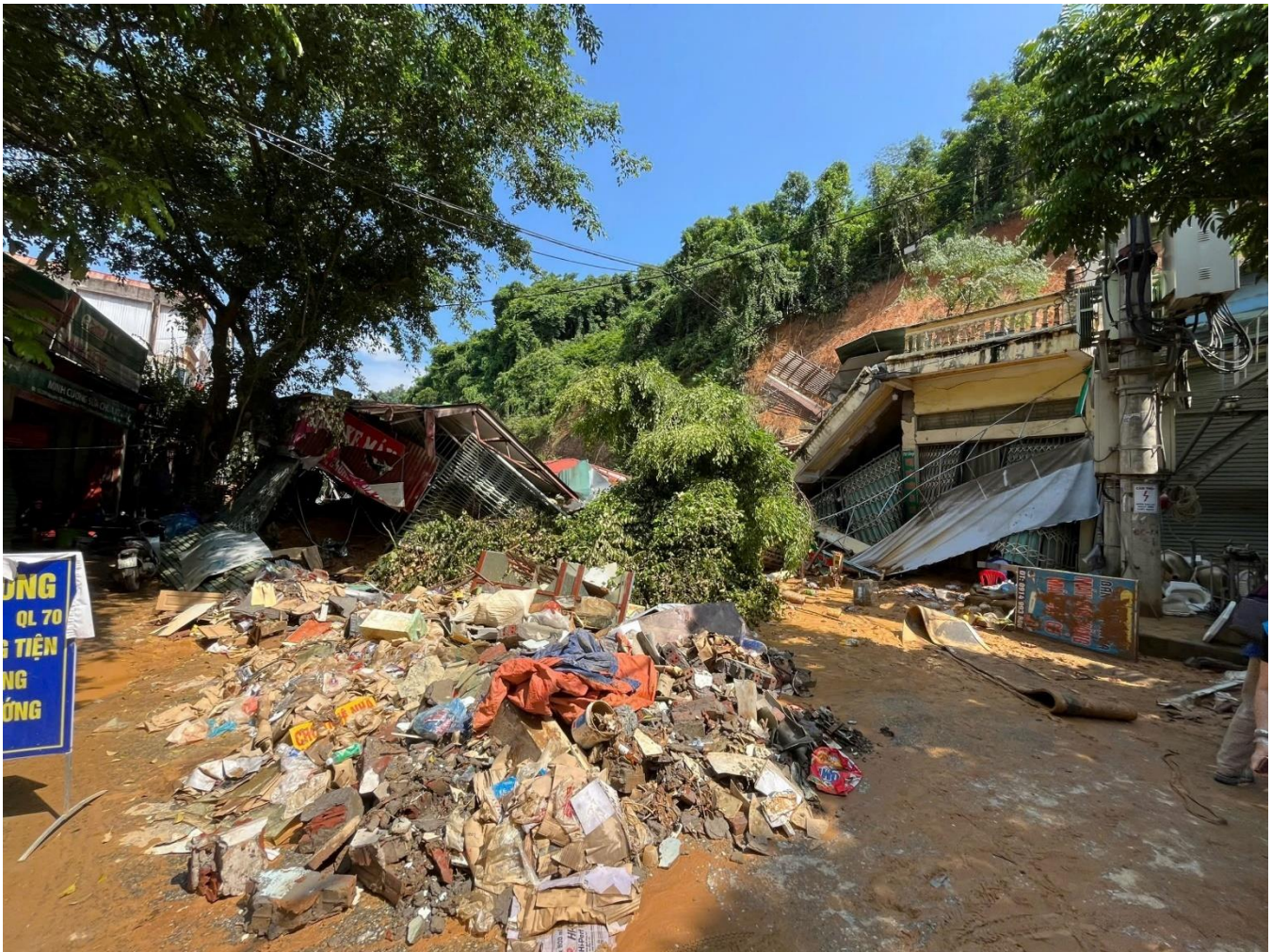
House damaged in Tran Yen district, Yen Bai province. Photo: UNDP
