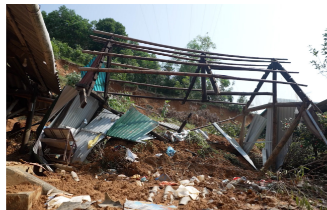
House damaged in Yen Bai province. Photo © UNDP in Viet Nam
