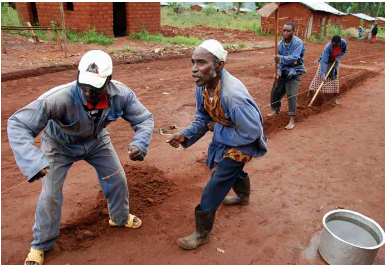
Local volunteers work together to build a road for their community in Burundi (UNDP Burundi/Aude Rossignol, 2013).
