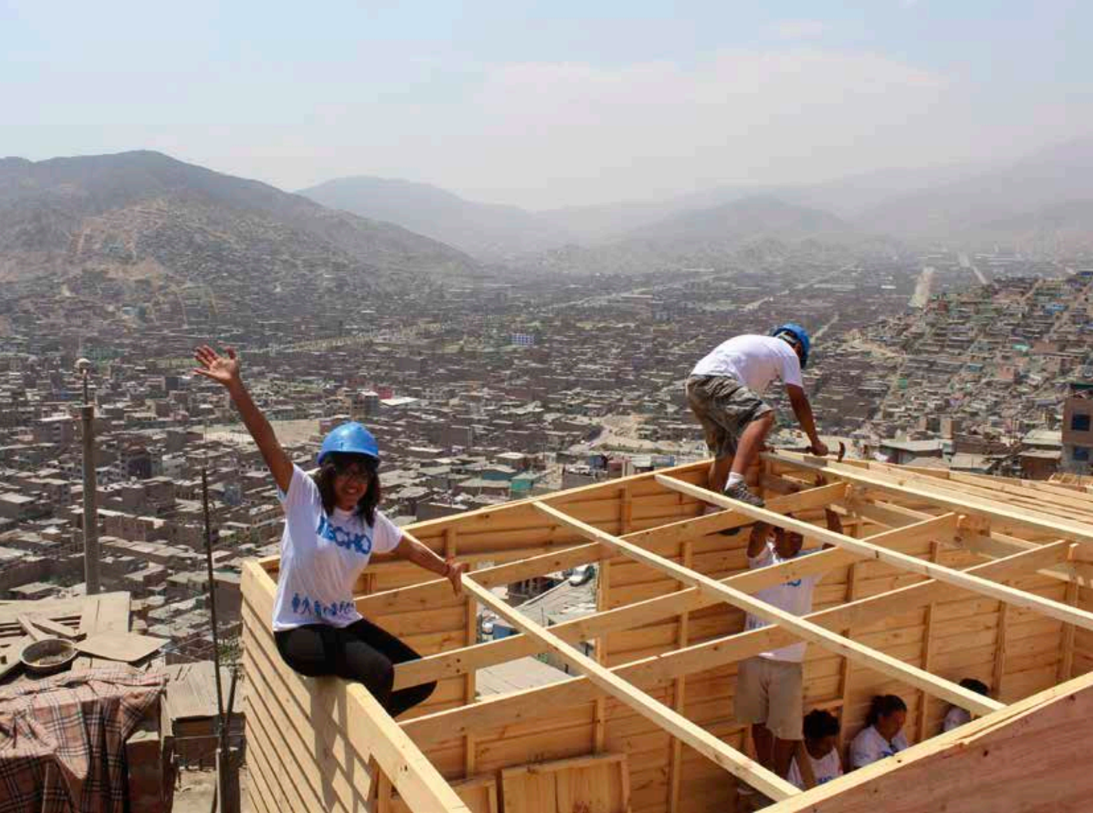
Techo youth volunteers work with urban communities to improve housing in Peru (Techo, 2017).
