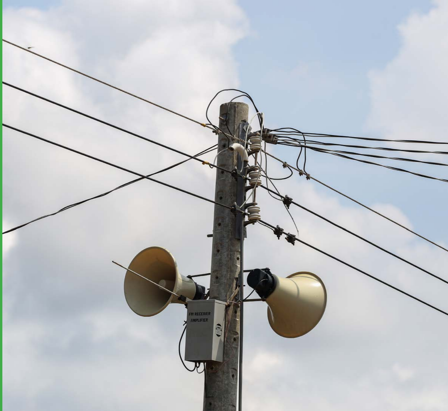
A broadcasting system in Soc Trang province, used to transmit messages to the community in an emergency. ©2015 Giang Pham/CARE
